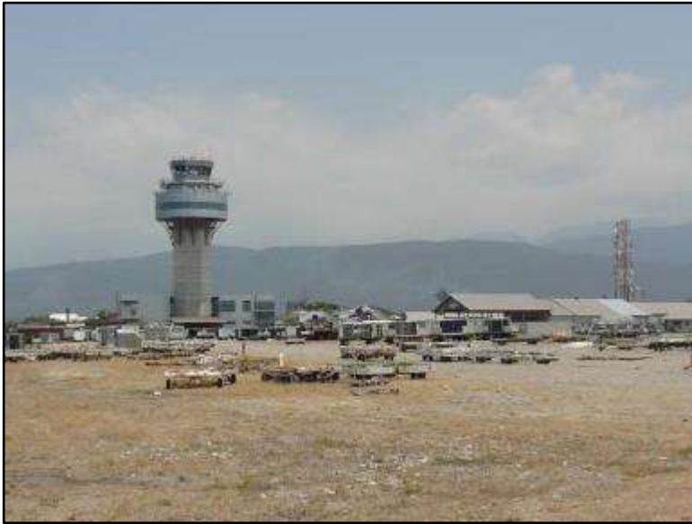
Figure 4.14 Airport equipment haphazardly stored in area behind RFFS
