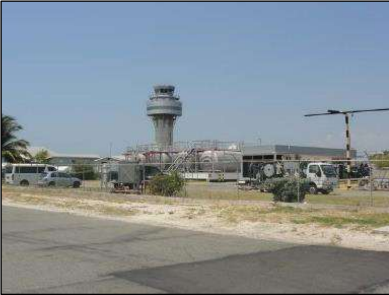
Figure 4.11 Fuel storage tanks in Fuel Farm
