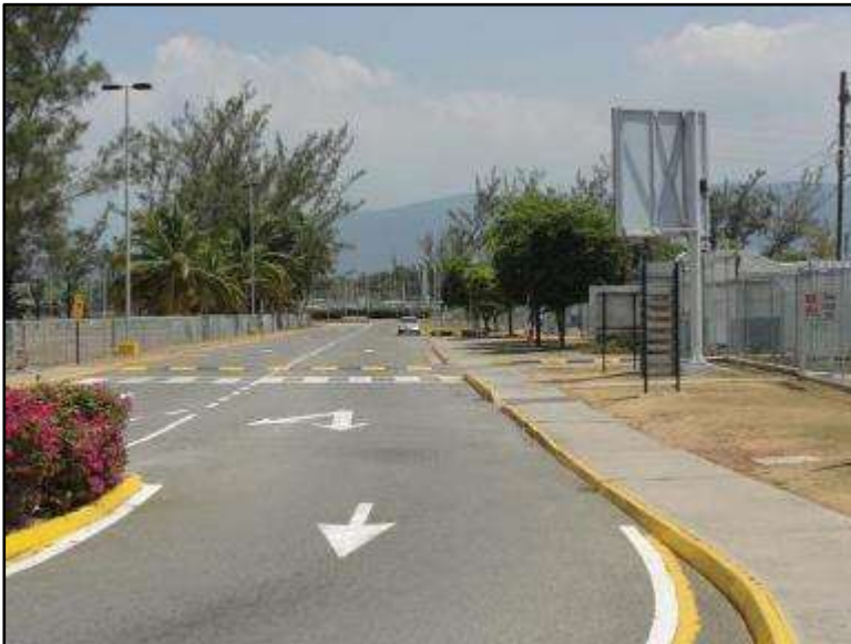
Figure 4:9 Two-laned Terminal Road leading to Departures and Arrival areas
