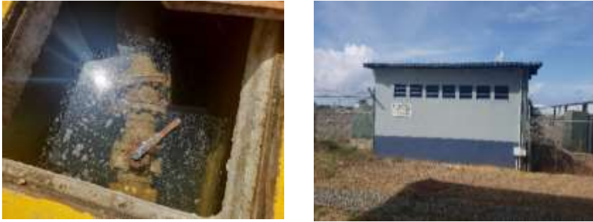
Figure 2.3 Samples of the pictures collected for the supporting buildings, substations and variety of pipes found across the airport property.
