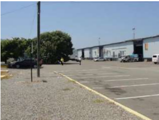
Figure 4.15 Landside access to Cargo Pier adjoining Terminal
