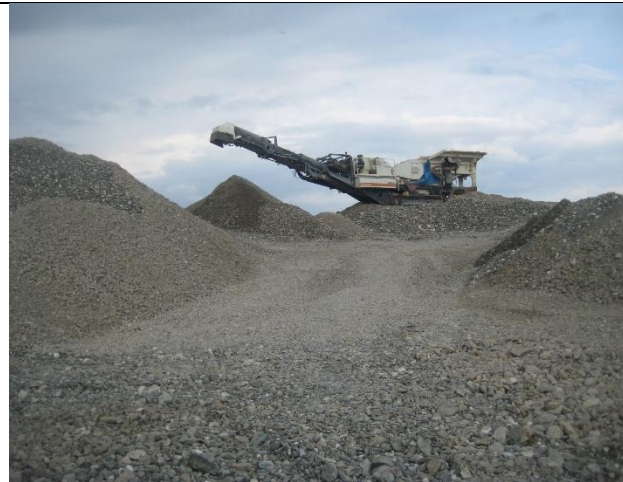
Plate 2.7. Crusher actively cutting stones. Crusher cutting stones too small.
